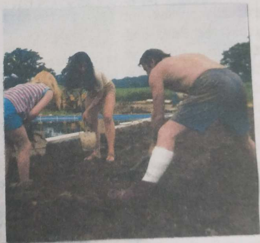
Tony Bowyer and family backfilling
